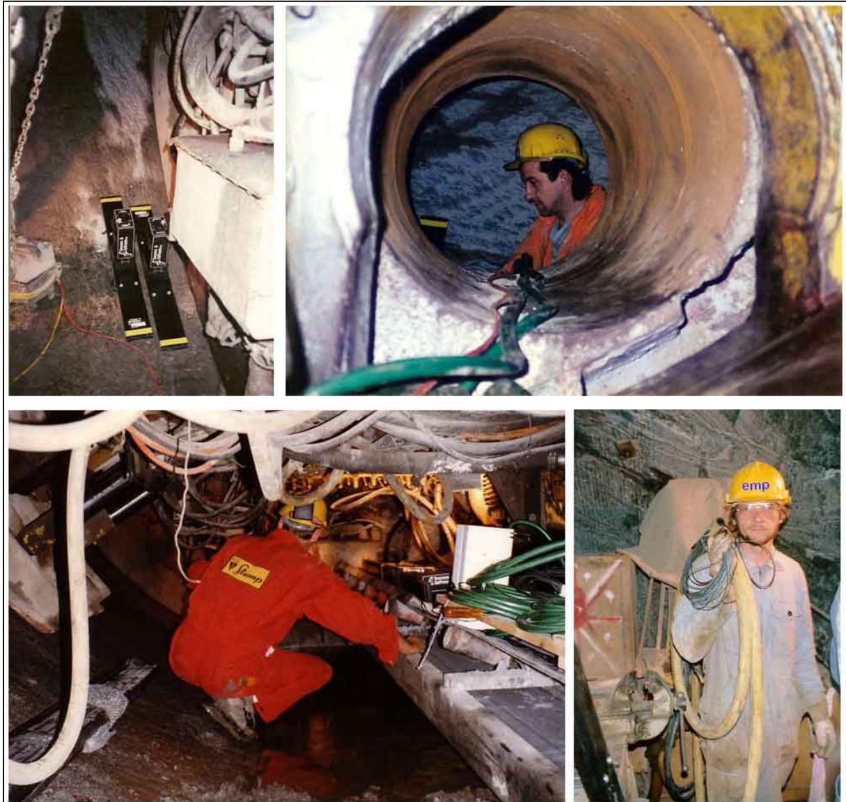
Fig. 6: GPR 100 MHz antennas (top left), Manhole with fibre optics (top right), engineers passing GPR equipment through a manhole (bottom left) and carrying protection tubes for the vulnerable fibre optics (bottom right). Photos: E Meier, U. Sambeth.
