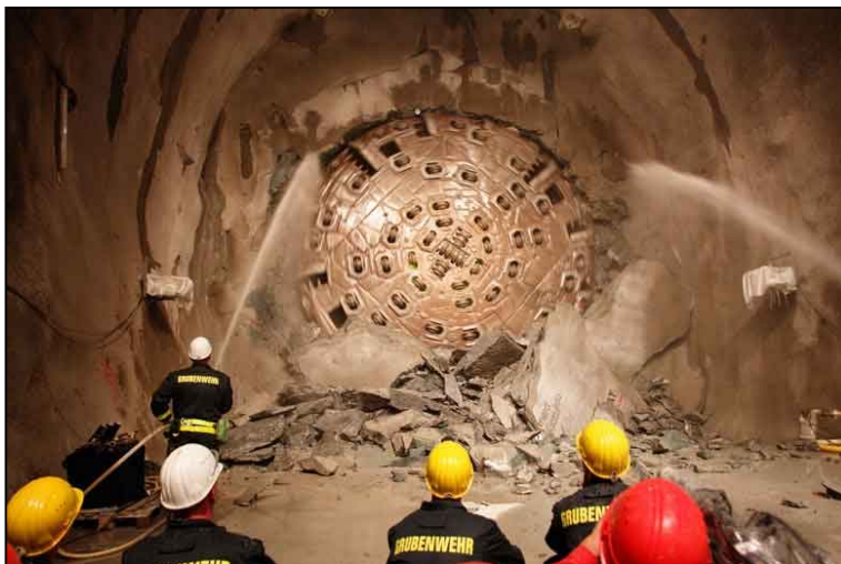
Fig. 2: Cut-through of the TBM on 15 October 2010.
