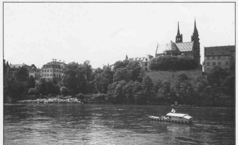
The slip zone is on the left of this picture, on an outer bend (left bank) of the Rhine in the centre of Basle. As the first course of action, granite blocks were placed on the river bank to stabilize the zone.
